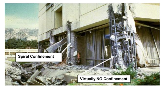
Circular spirals confine concrete far more effectively than one-dimensional ties. The helpful effects of circular spiral steel reinforcement embrace strength sweetening, a rise in strain admire most strength, and a greatly exaggerated ability of the concrete to sustain giant deformations while not vital strength loss. once concrete sections square
